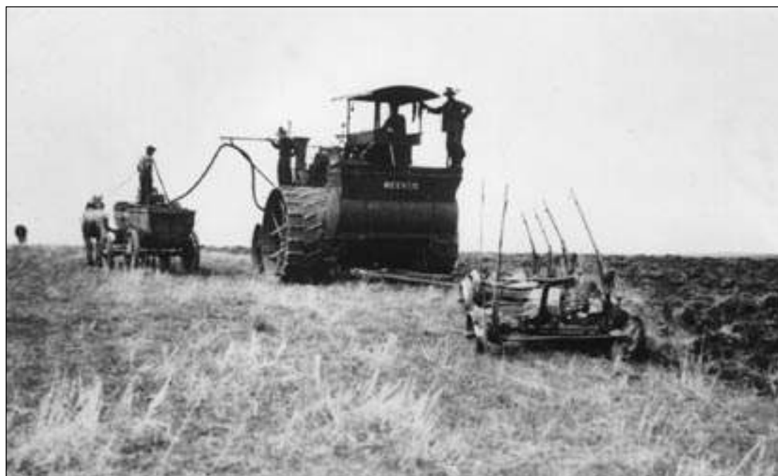
► Breaking land at Standard. A water wagon is behind the Reeves steam engine, replenishing its water supply. (c. 1920)
