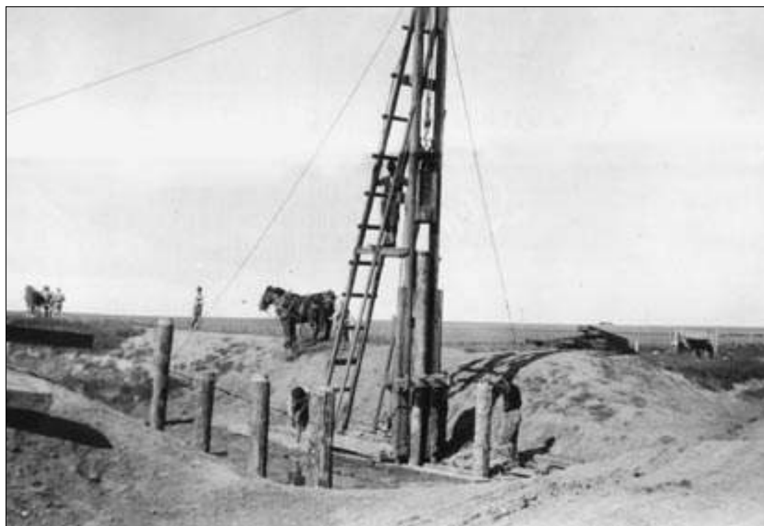
► A horse powered pile driver on the main irrigation canal in the Monarch area of the Eastern Irrigation District. (c. 1922)
